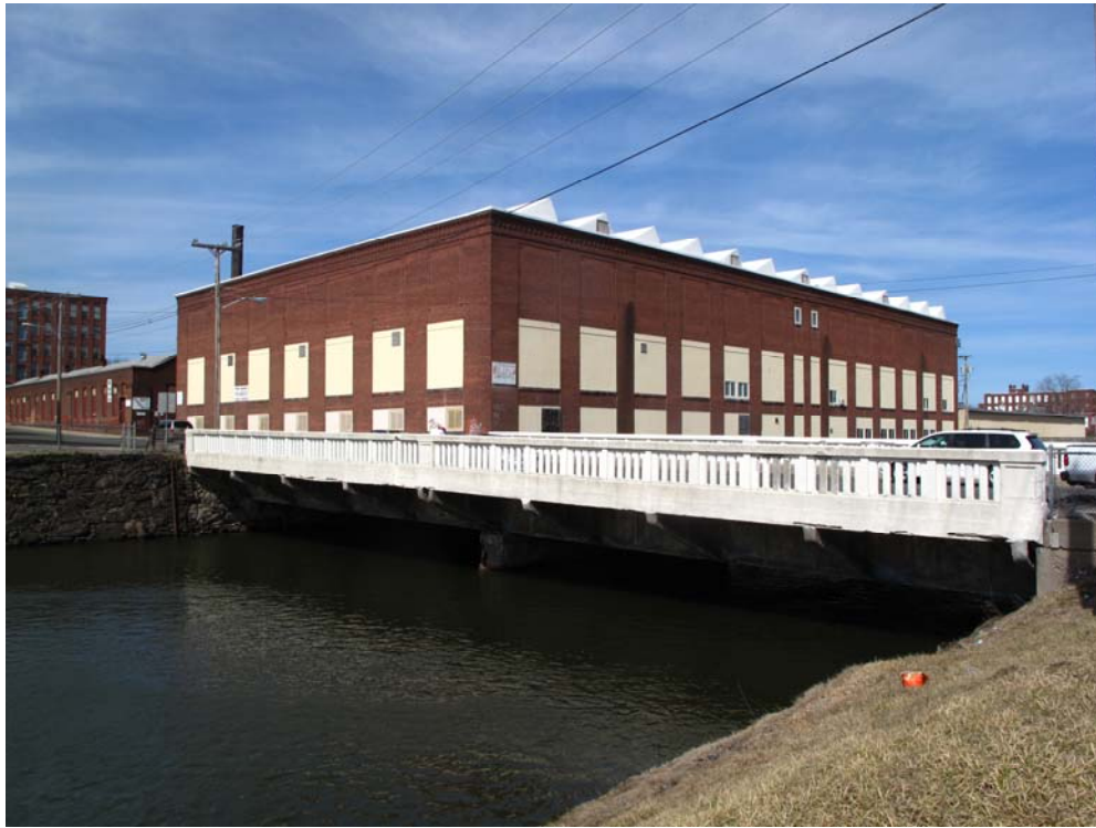
Figure 10. View from south over Second Canal. (by author)
